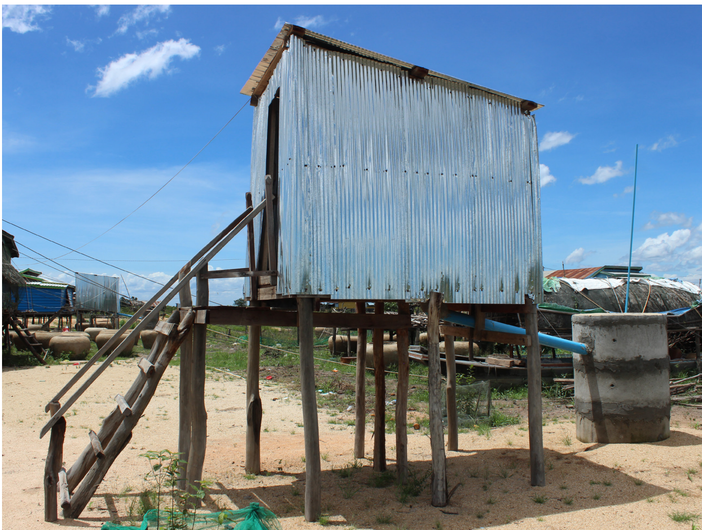
An elevated latrine in flood-prone Trapeang Chan commune, Kampong Chhnang province, Cambodia
